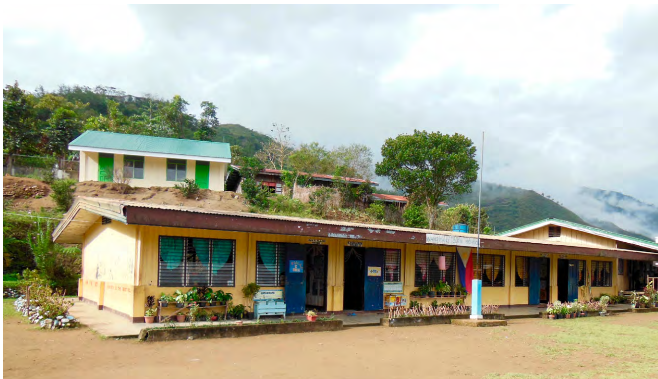
The school building in the community of Binablayan, Tinoc. Photo credit: Pernilla Malmer
